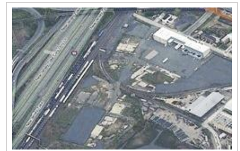
The complex site spanned two municipalities and was constrained by roads, rails, and wetlands
