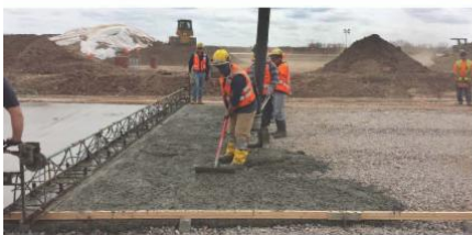
Workers lay foundation for the new 700-megawatt natural gas-fueled power generation facility constructed by Competitive Power Ventures.
