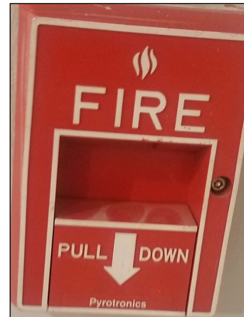
Pull Stations with Pull Handles Only
