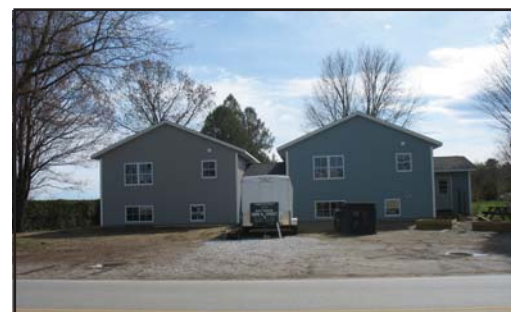
Habitat for Humanity's new duplex on the former Litchfield property, with construction nearly complete.
