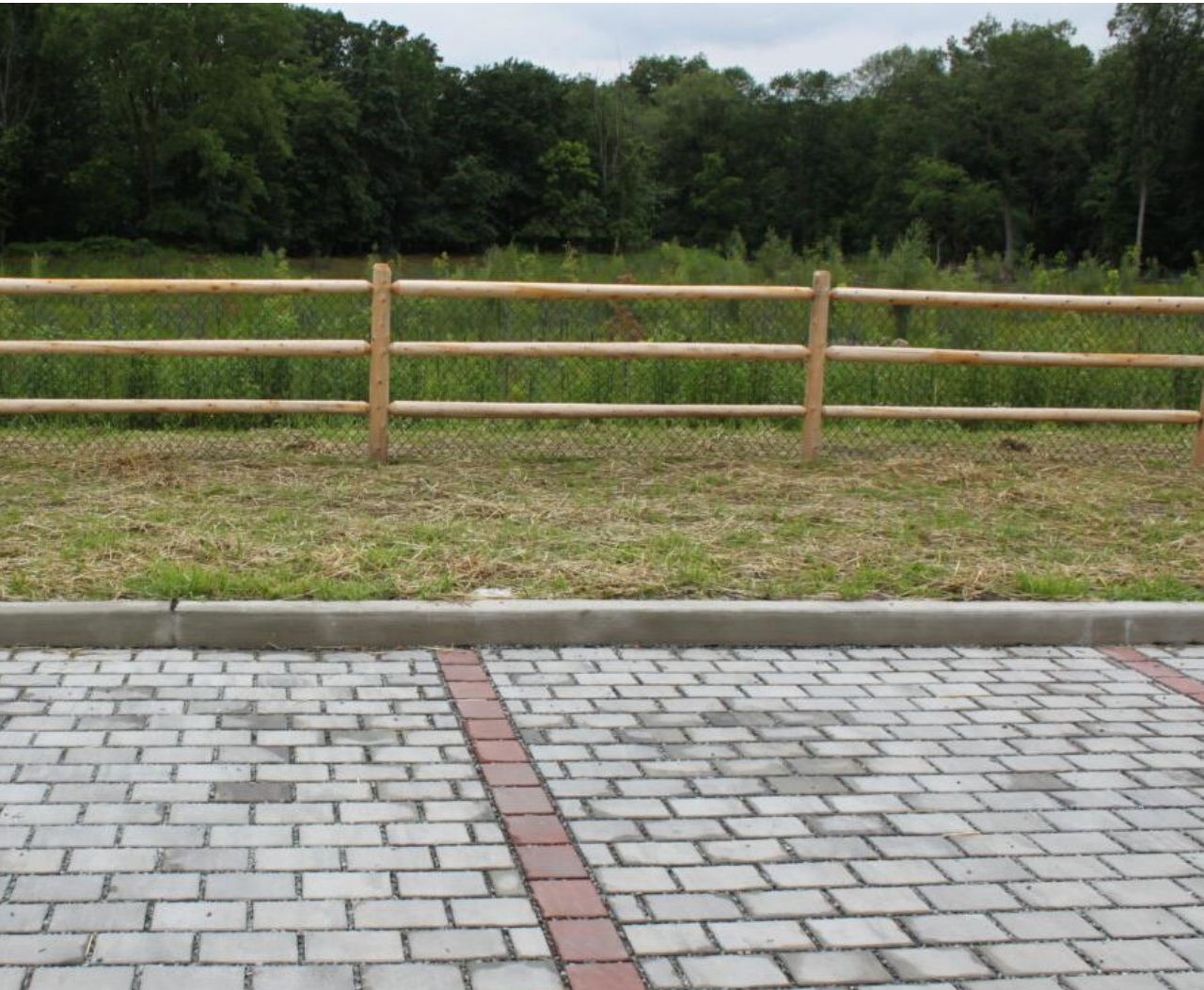
Permeable Pavement in Bloomfield, NJ
