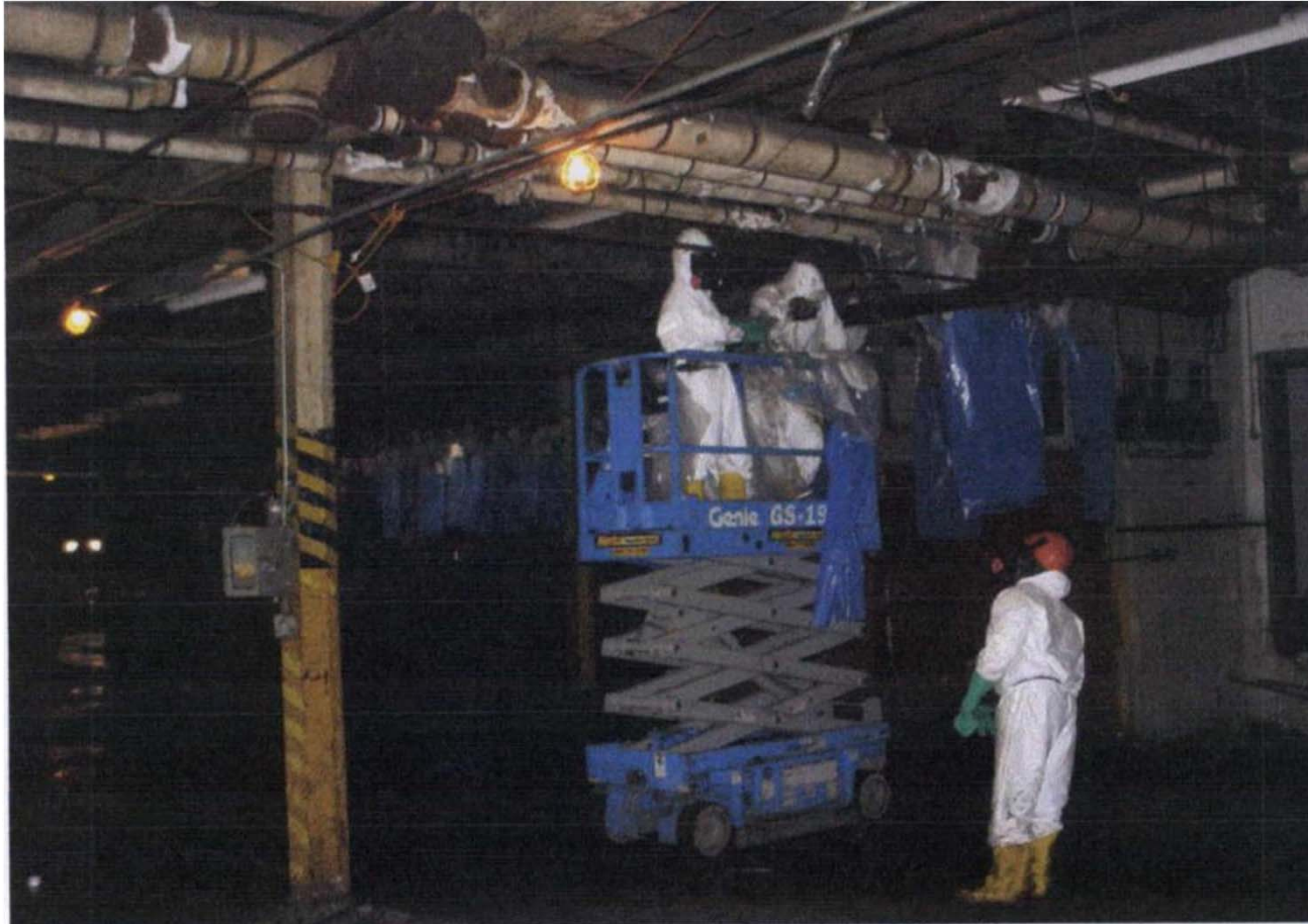
View of ACM pipe insulation removal at Building #1- 1 st floor.
