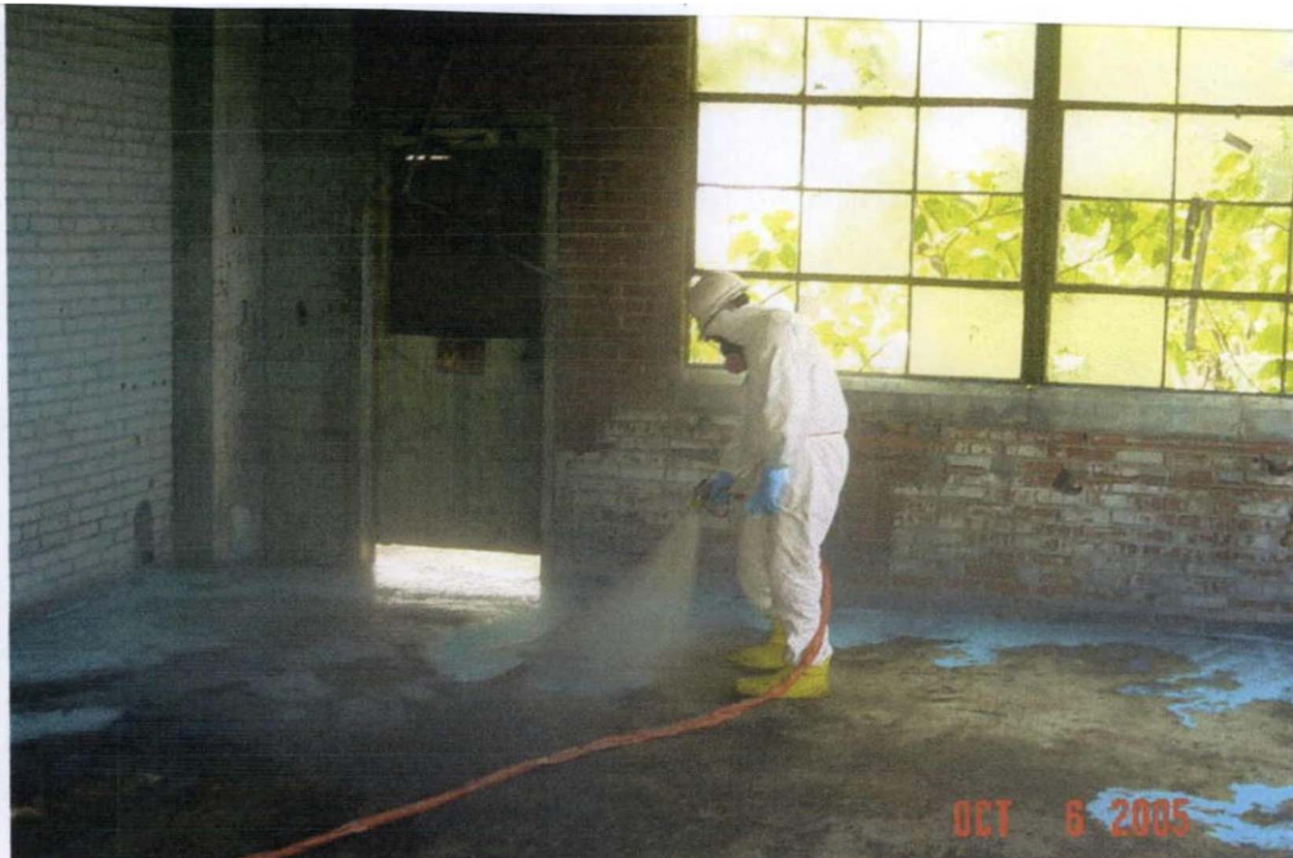
View of sprayed-on ACM encapsulant application activity at Building #2- 2 nd floor.
