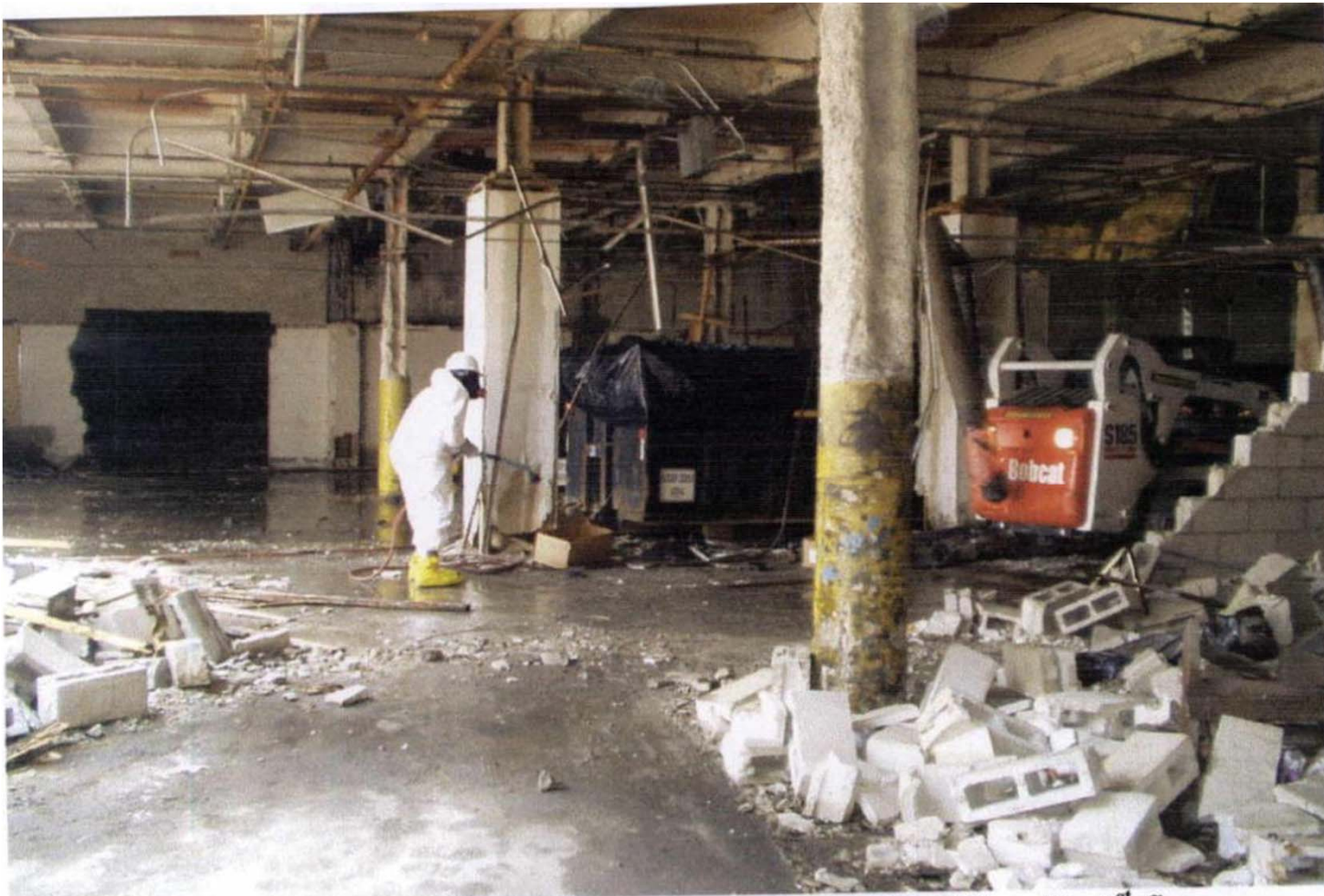
View of ACM debris/ concrete block removal activity at Building #2, 1 st floor.
