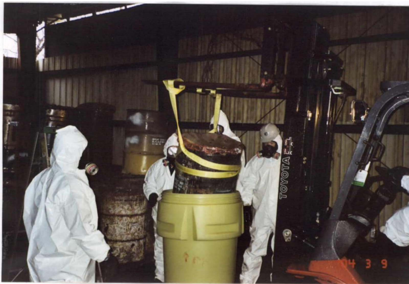
Picture No. 17 - Earth Tech personnel overpacking drum of high pH material in the Waste Storage Building
