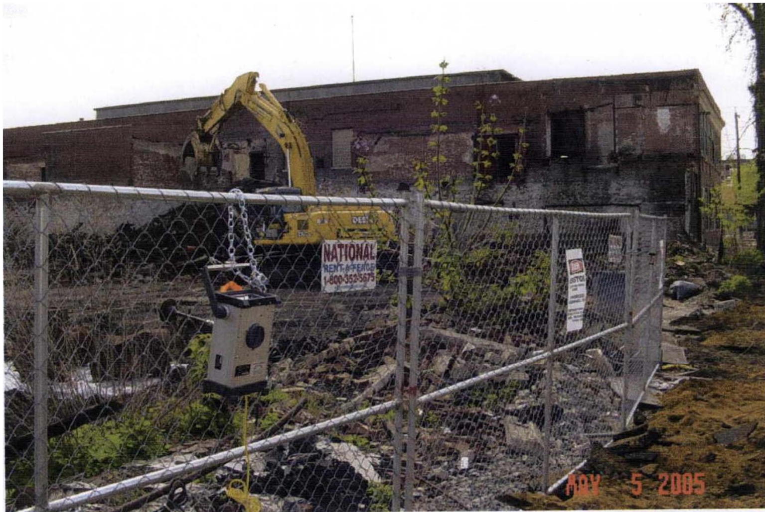
View of perimeter air monitoring station at west fenceline.
