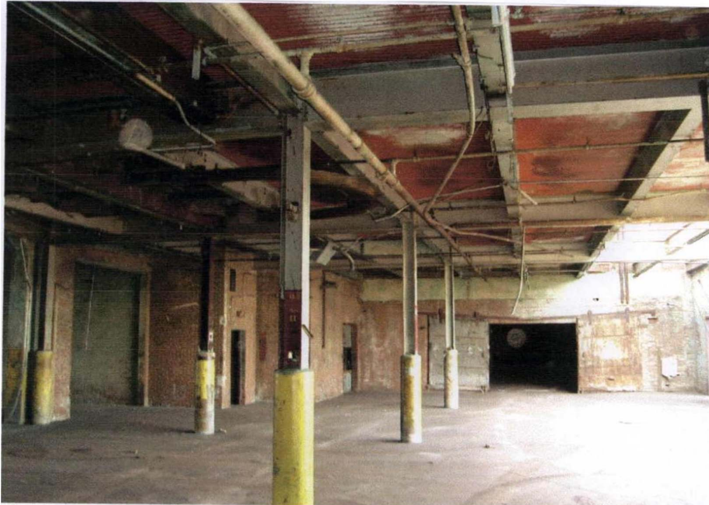
View of completed decontamination and ACM encapsulation activity at Building #2.
