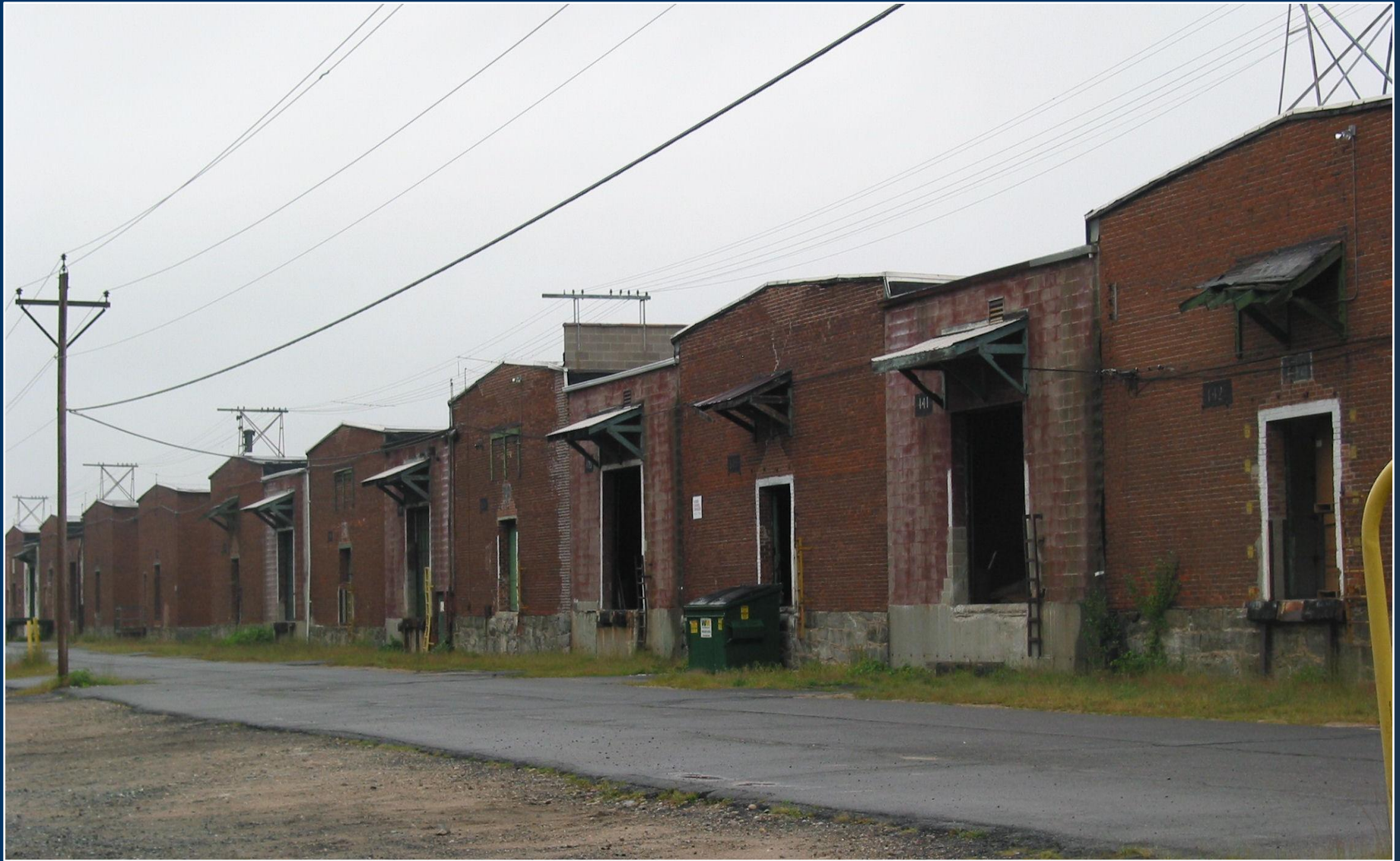
Stockhouses looking West
