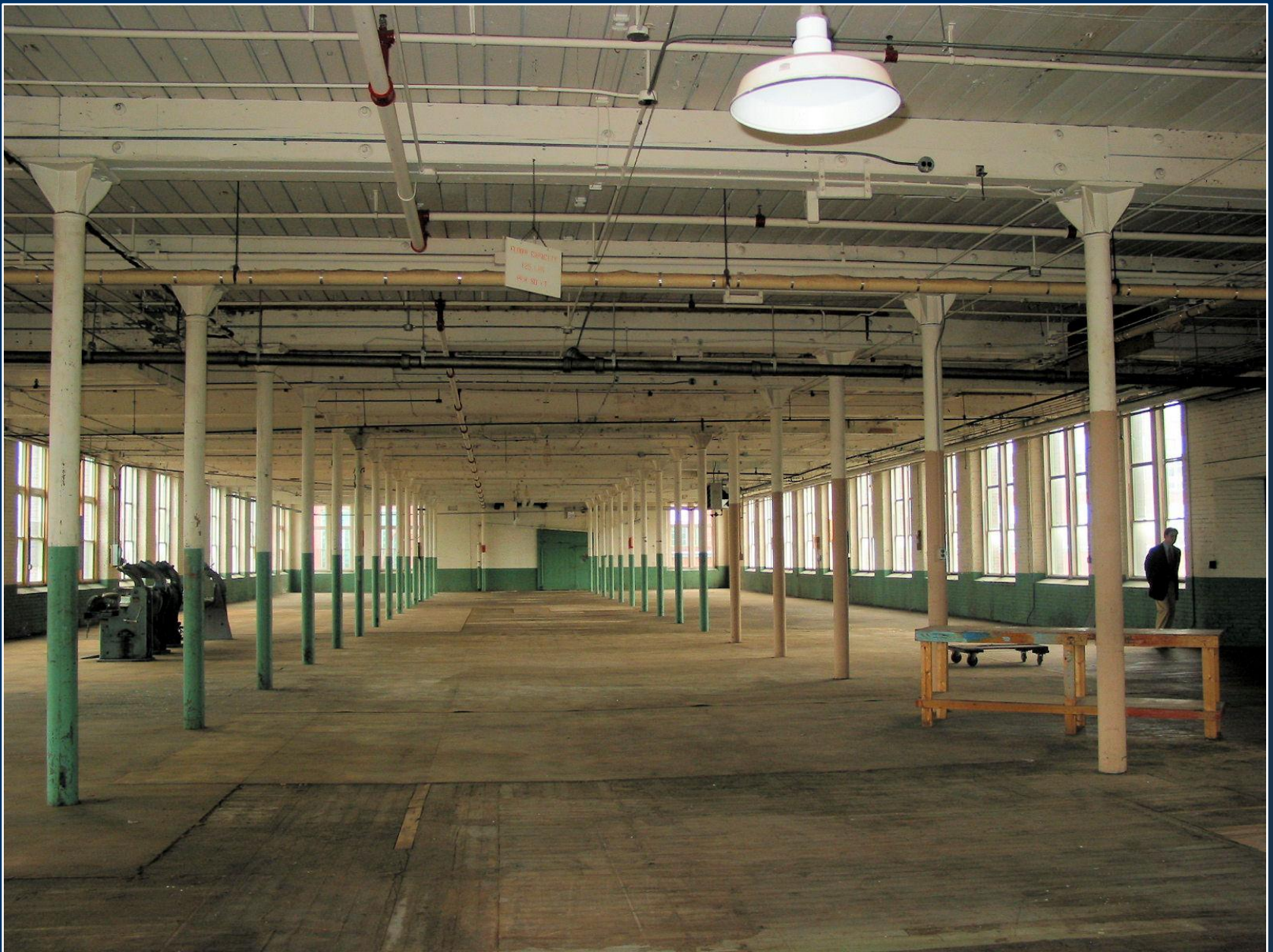
Building 8 Addition 3 rd Floor
