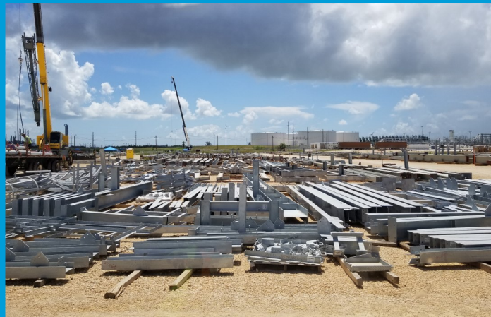
An on-site storage and laydown facility.
