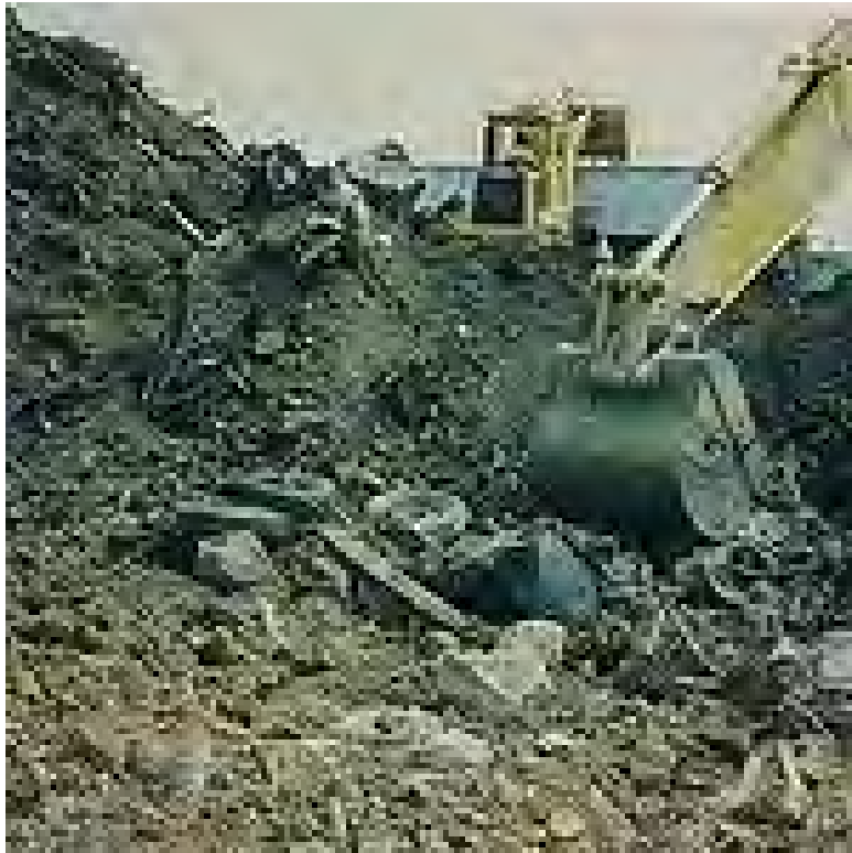
Landfill During Excavation
